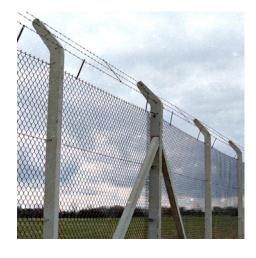
Chainlink fencing is made from galvanised wire and then plastic coated, and woven together to give a strong and cost effective way of fencing.
